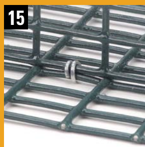
Cage grid secured with a blunt 15-gauge C-Ring.
