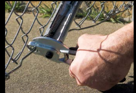
HFP9 Attaching tensioning wire to chain-link fence with 9 gauge aluminum hog rings
