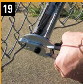
HFP9 Attaching tensioning wire to chain-link fence with 9 gauge aluminum hog rings
