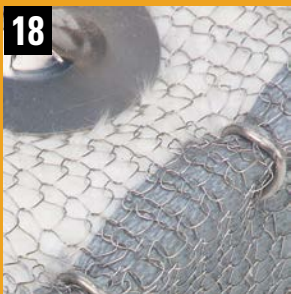
Heat and sound insulation stitched with 16-gauge stainless steel C-rings.
