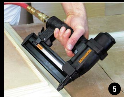
18-gauge brads applying trim
